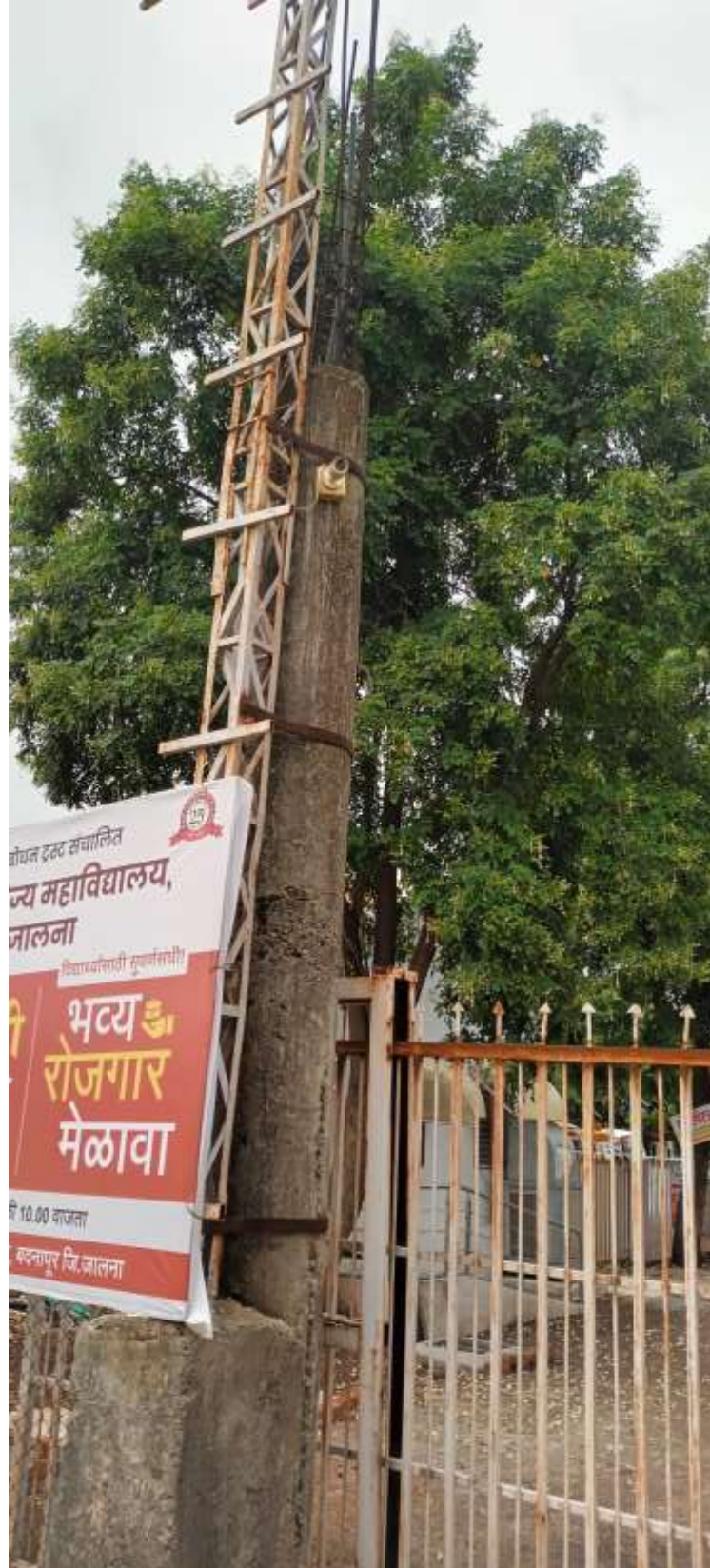
CCTV CAMERA AT ENTRY GATE OF CAMPUS
